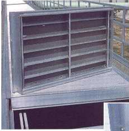
Figured above: A panel covering affluent channels is removed to show its relative size. The panel measures 3.5' x 6'.
