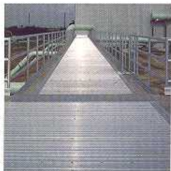
Pictured above: This portion of the cover stretches over effluent channels and measures more than 150 feet. It is composed of a series of interlocking panels sealed with neoprene gaskets (see back of flyer for detail).
