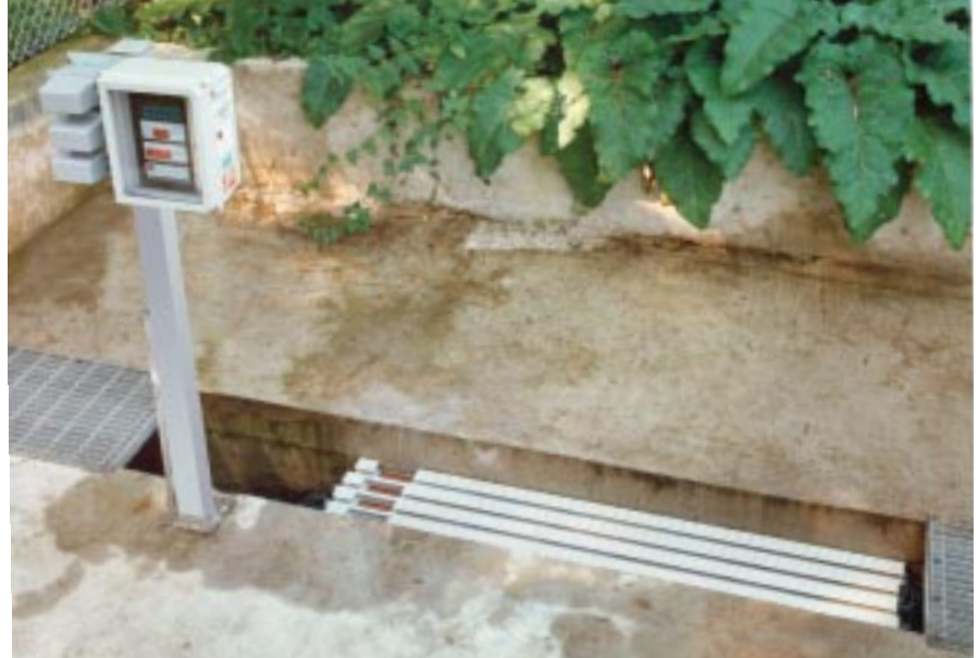
The Trojan UV3000™PTP system delivers flexibility and cost savings through its simple installation in existing channels and chlorine contact tanks. The system is completely stand-alone and can be situated outdoors with no additional building, shelter or cooling requirements.
